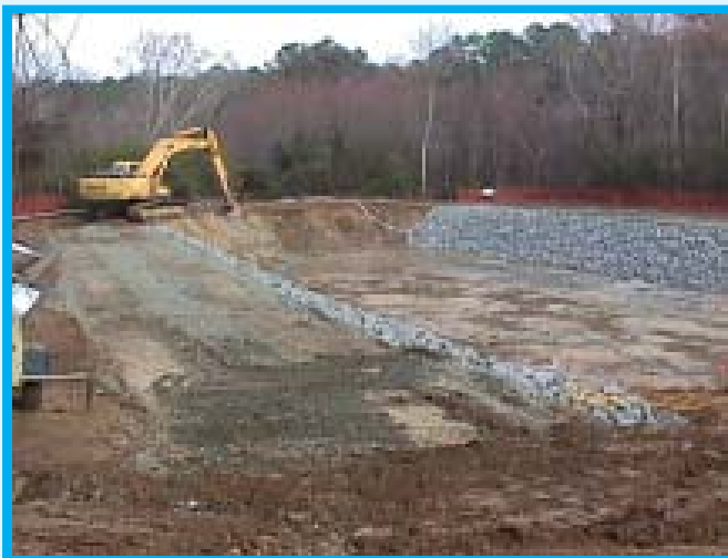
ORIGINAL FOREBAY CONSTRUCTION (2001)
